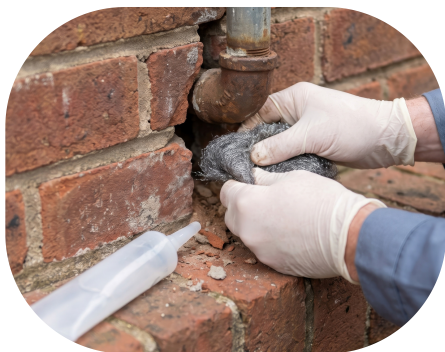
Pack utility voids with stainless mesh and seal tightly with outdoor sealant.
